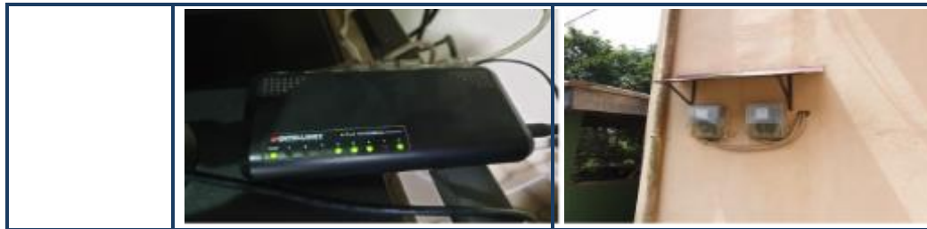
[Figure III-24] Rathnapura District Survey Office
