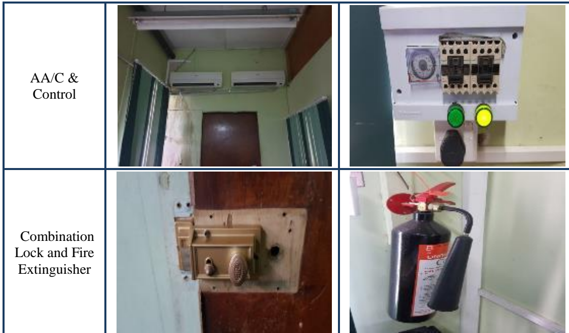
[Figure III-18] Old Server Room Environment Facility
