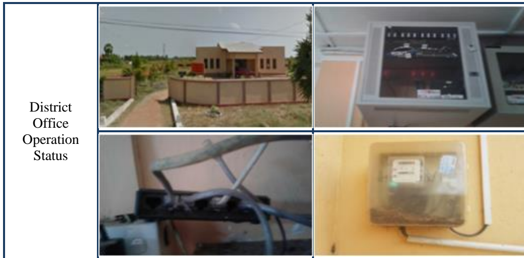
[Figure III-42] Mannar District Survey Office
