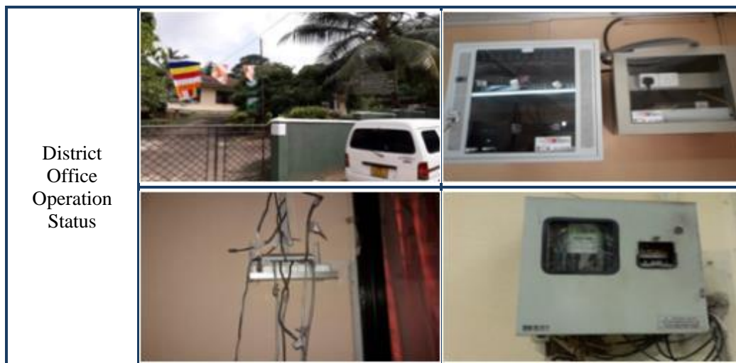
[ Figure III-34] Kegalle District Survey Office
