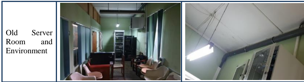
[Figure III-13] Environment of Old Server Room and Interior
