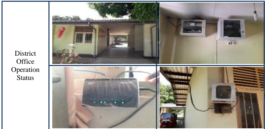
[Figure III-26] Polonnaruwa District Survey Office
