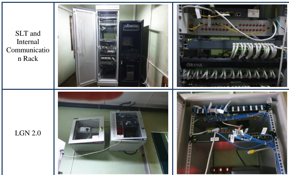
[Figure III-16] Network Facility Rack
