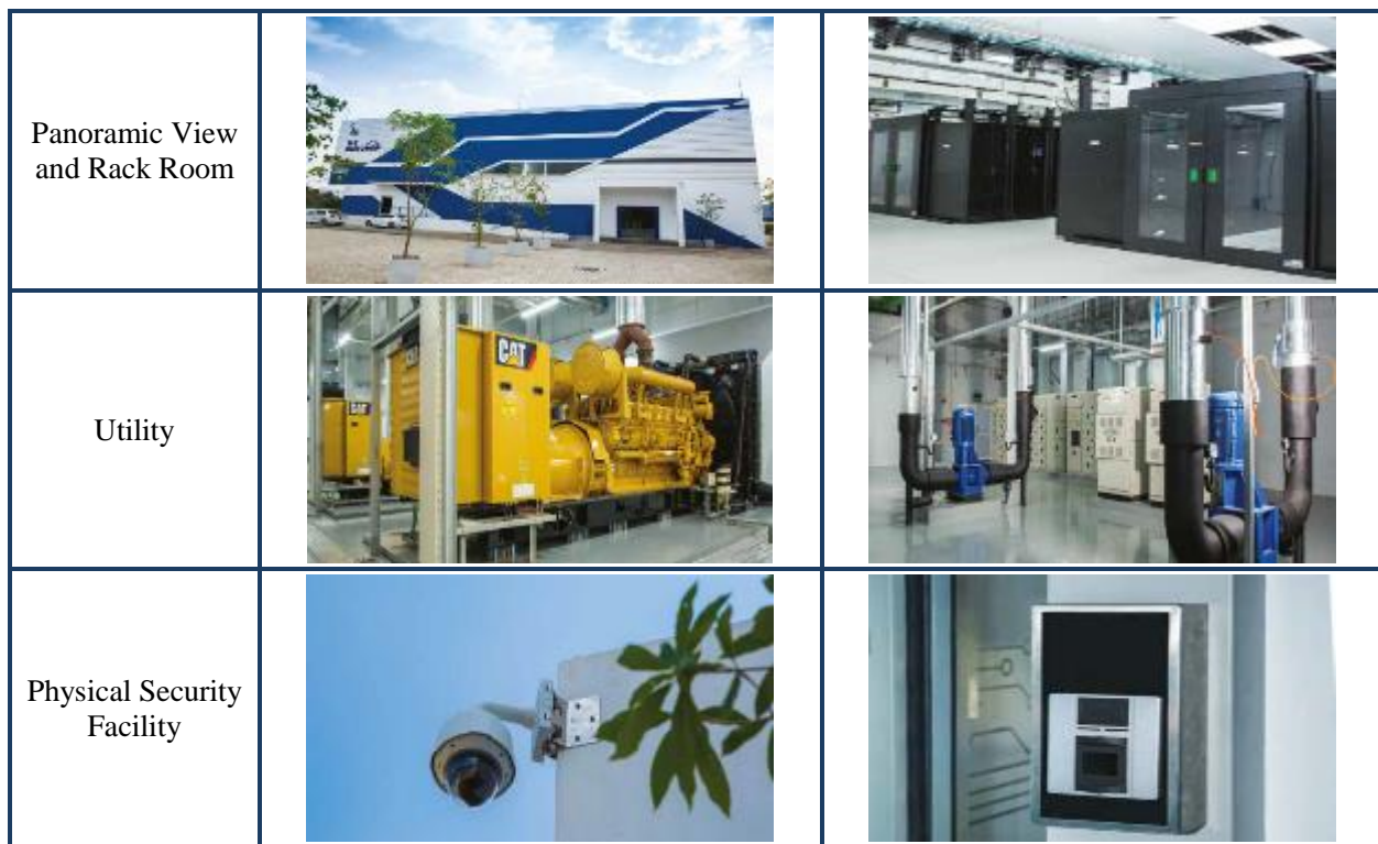
[Figure III-47] SLT IDC Facility Status
