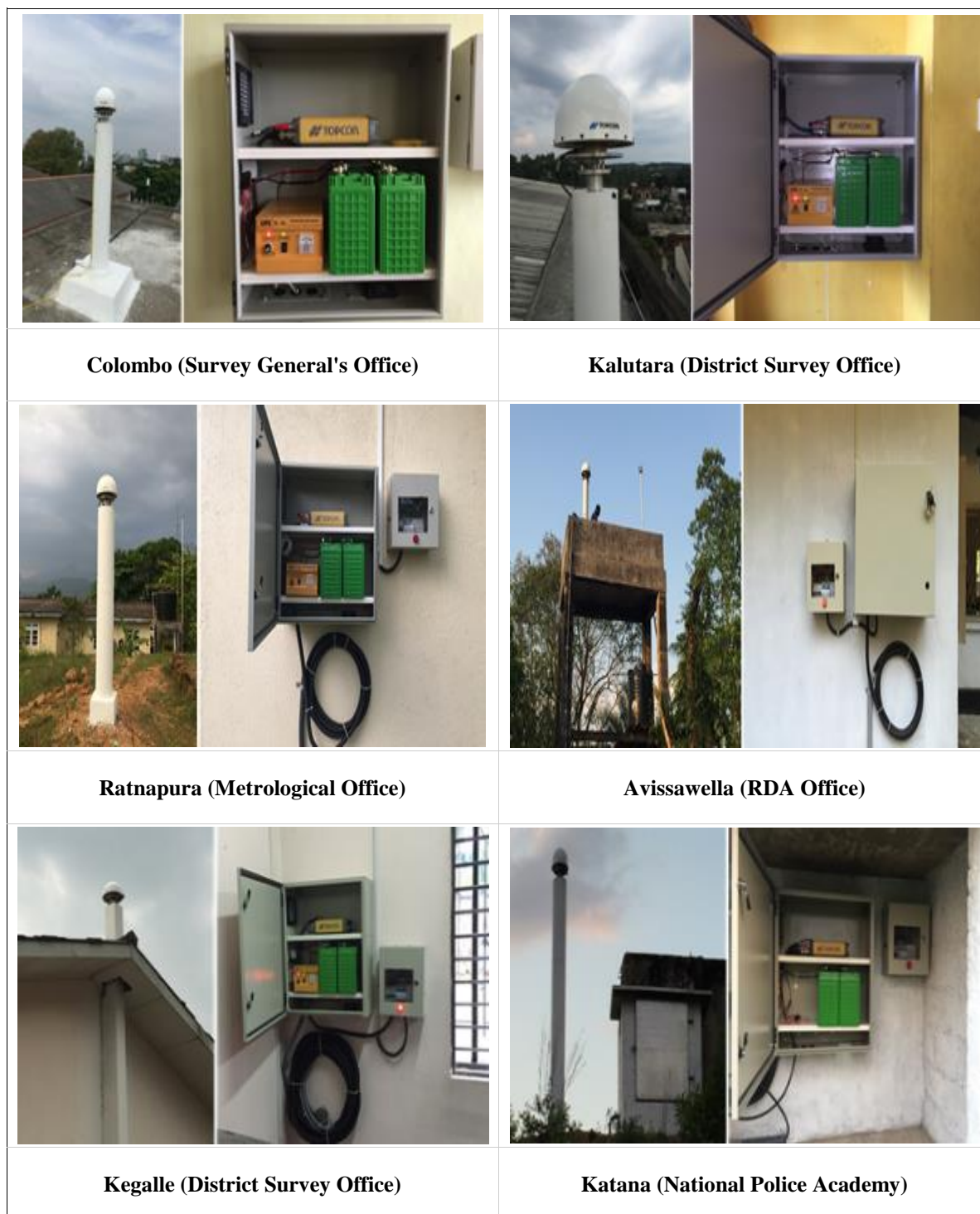
[Figure III-4] CORS Installation Status
